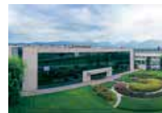
The New Factory
