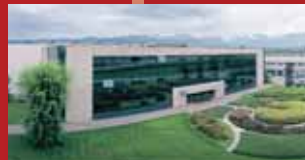
The New Factory
